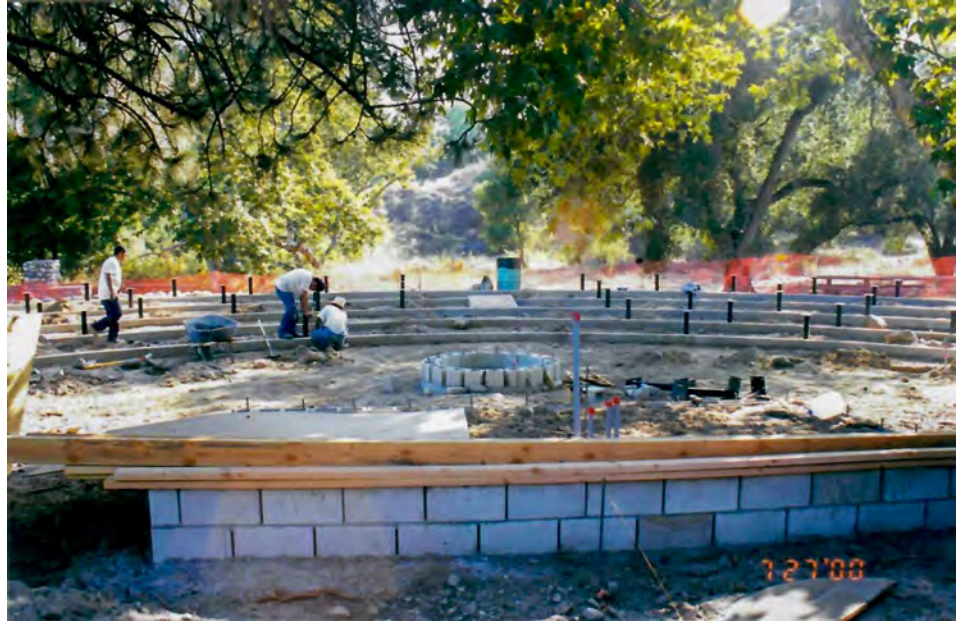
Original construction of outdoor classroom - 2000
